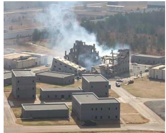
Figure 4 - Chemical Plant Explosion and Collapse
